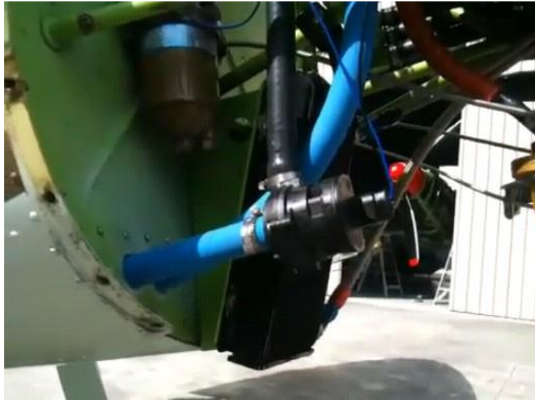
Figure 6.5: Installation of a 15 L/min booster pump
